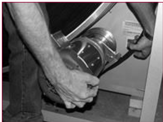
Belt being removed from the motor sheave.
