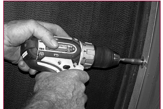
Loosening of Tek screws prior to seal adjustment.
