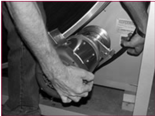
Belt being removed from the motor sheave.
